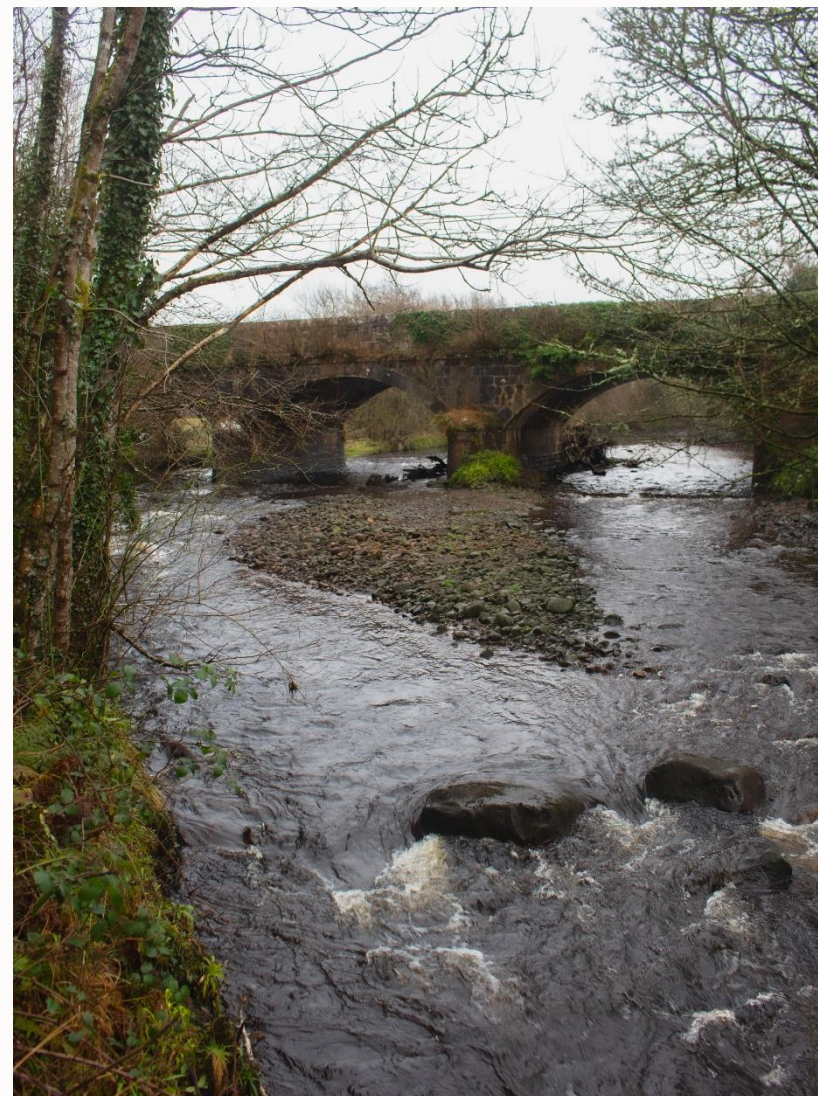
Figure 23. Yellow River and Owenboy bridge
